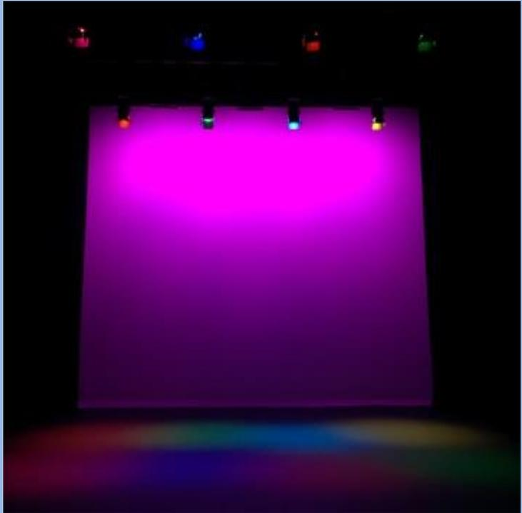
**Photo: The new Dunamaise stage lighting with 2kW of LED lamps replacing 24 kW of standard stage lighting.**
