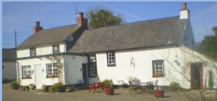
Photo: Econcertive Home Base at the start of project.
